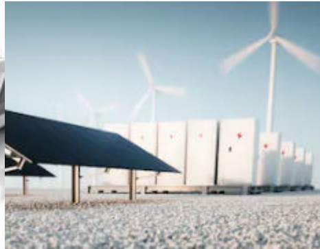
Energy Storage System
