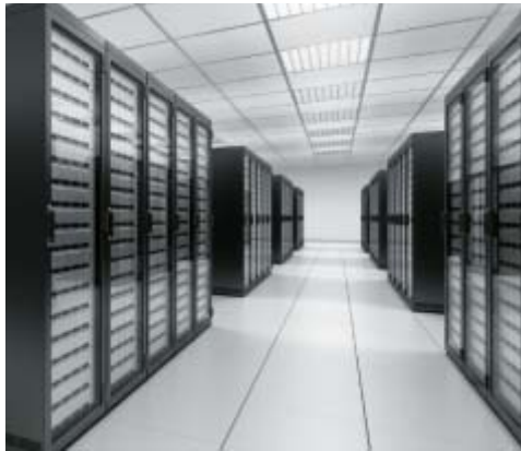
Cooling Module in Cloud Computing
