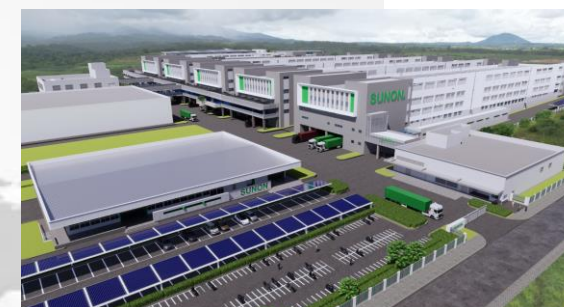
Bataan, Philippines II (Under Construction / Conceptual Image) Fan & Module
